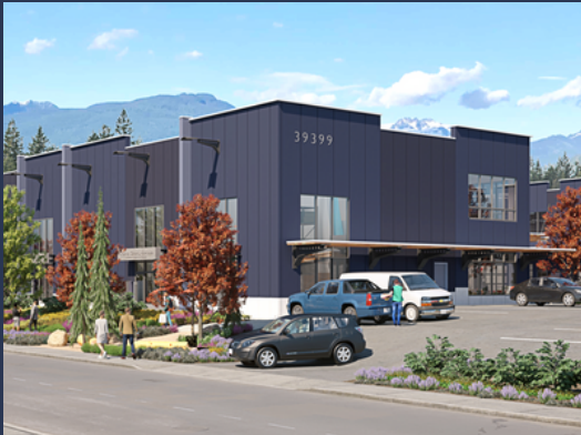
39449 QUEENS WAY, SQUAMISH
